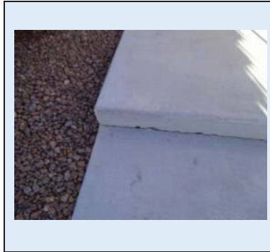
Settling Cracks @ Riser Joints for each of the front stairs.
